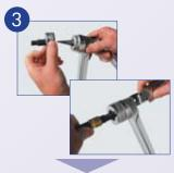
Expand the pipe using the PSC Expanding Tool making sure the jointing sleeve is well away from the area of pipe to be expanded. Expand the pipe twice to make a good expansion of the pipe end.
